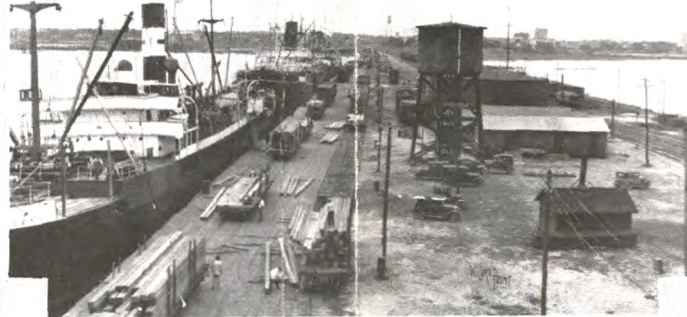
DEEP WATER PORT - GULFPORT
