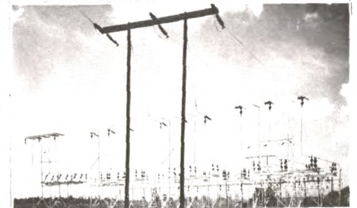
ELECTRIC POWER - GREENWOOD
