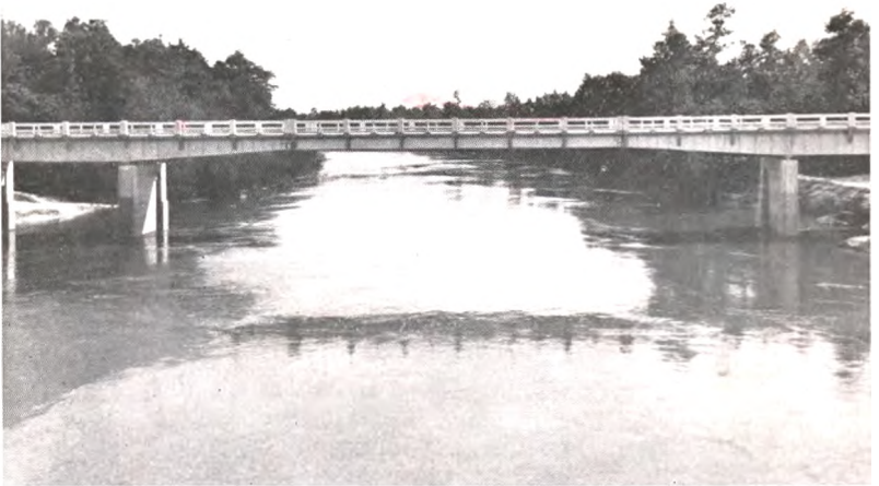
STEEL AND CONCRETE BRIDGE
