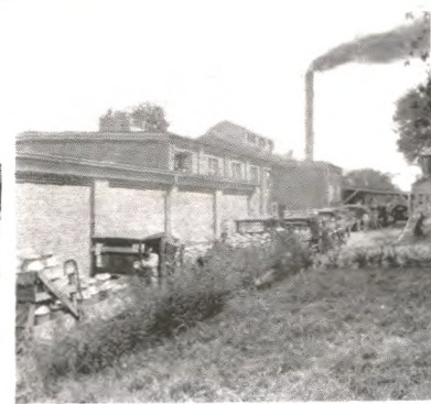
CONDENSED MILK PLANT STARKVILLE
