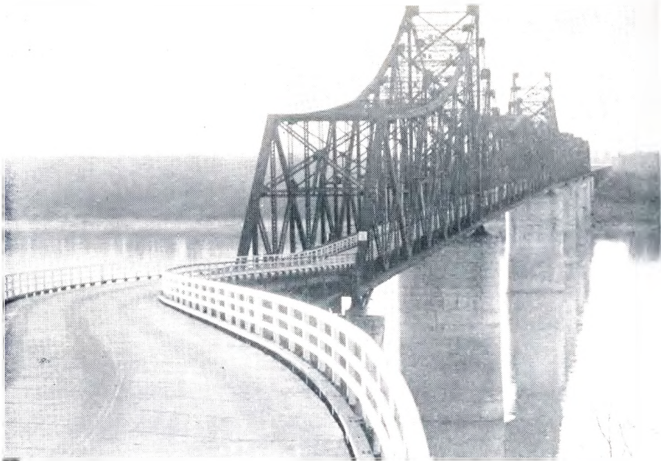
This Bridge spans the mighty Mississippi River at Vicksburg, Mississippi
