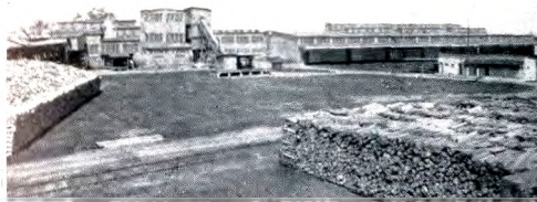
INSULATION BOARD PLANT - GREENVILLE
