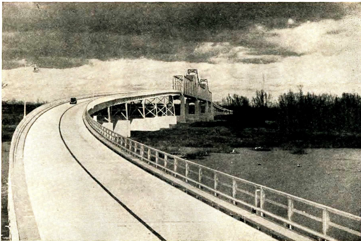
Greenville-Lake Village Bridge over Mississippi River
