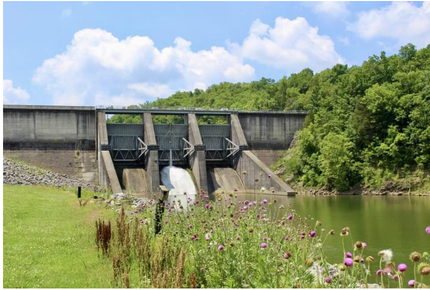
Figure 1. Tellico Dam (Photo by author)
