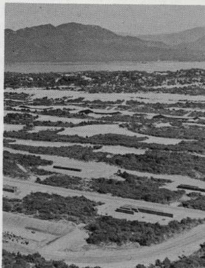
Stripping forms on foundations
