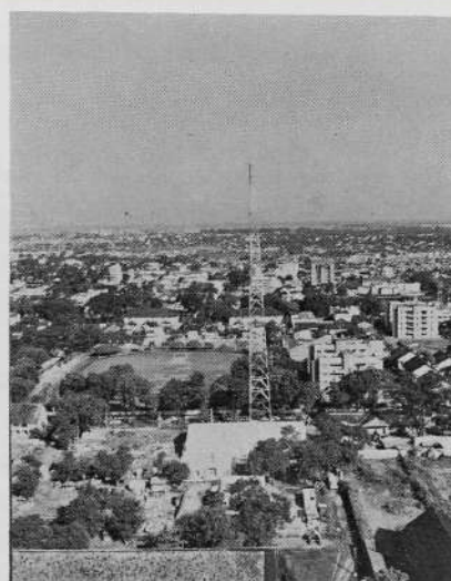
Downtown Saigon — Armed Services Radio and TV Studio and tower built by our client
