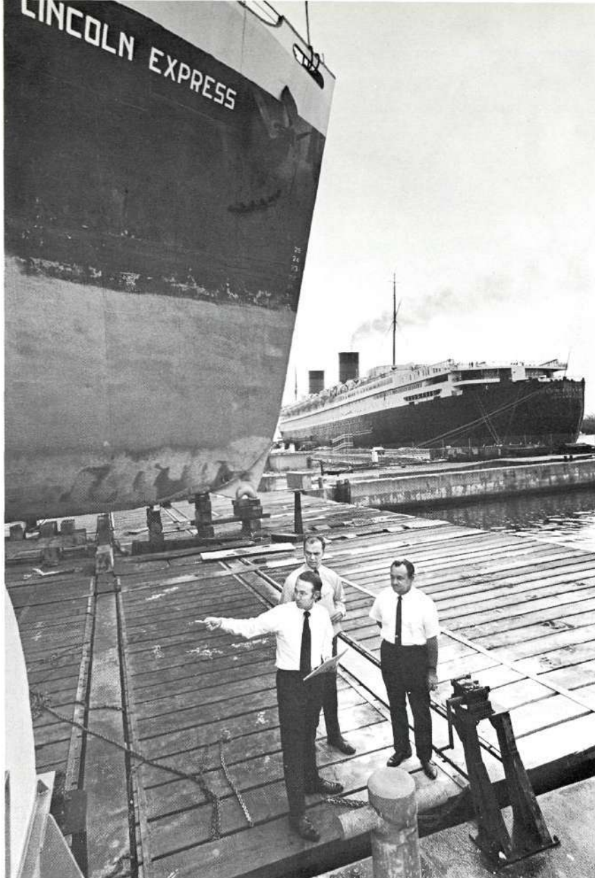
Port Everglades Shipyard operates a unique drydock equipped to lift huge ships completely free of the water for repairs and cleaning. With R. L. LaJoie, Jr., vice president (r.), are senior Bob Rives, in the foreground, and senior assistant Jim Rosemurgy. In the right background is the original Queen Elizabeth , moored at the port as a tourist attraction.
