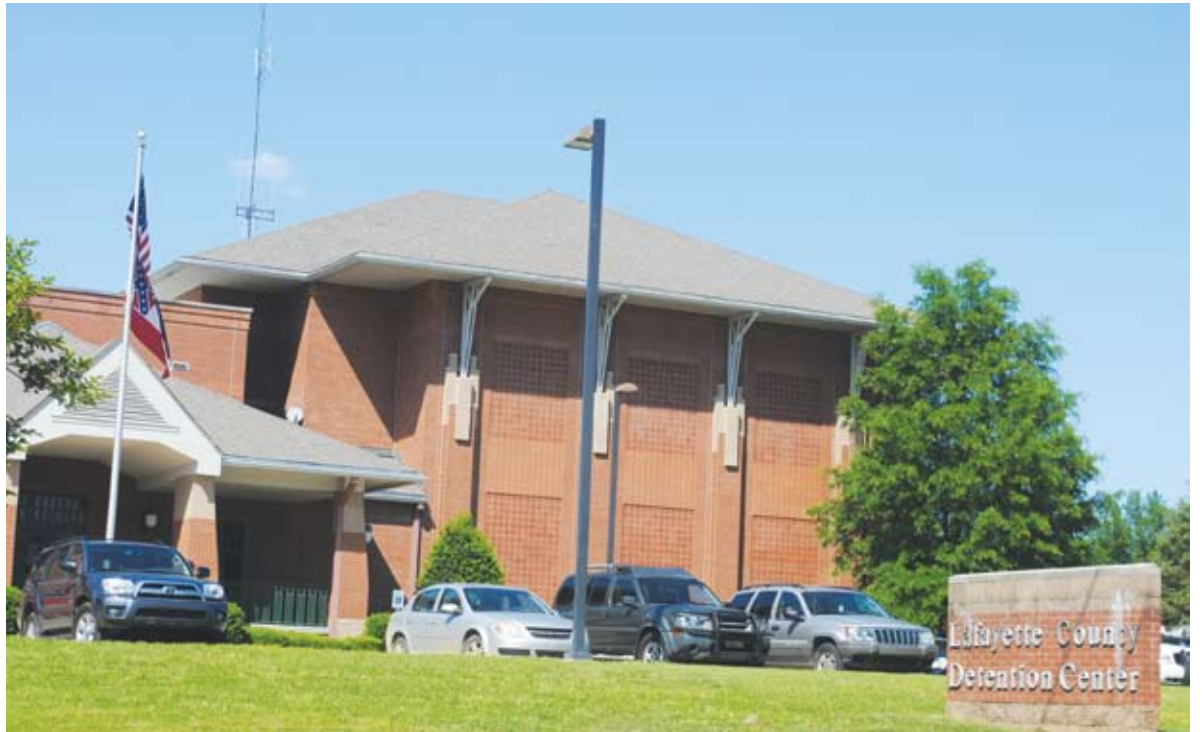
Lafayette County Detention Center
