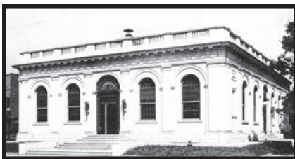
Federal Post Office Building circa 1913
