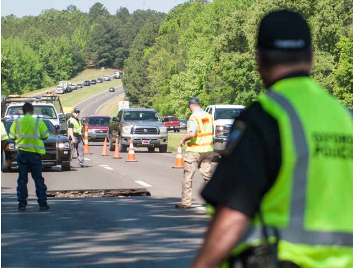
A sink hole on Highway 6 near Chucky Mullins Drive causes delayed traffic on Wednesday morning.
