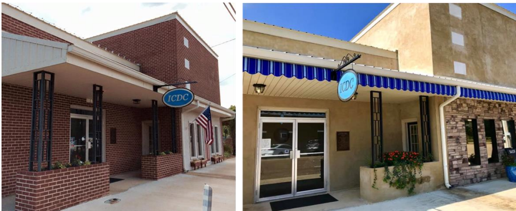
Figure 12: Itawamba County Development Council Building
