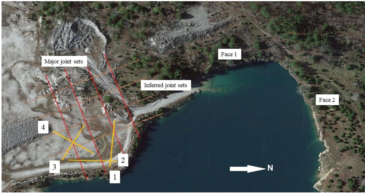
Figure 41: Observed joint system.
