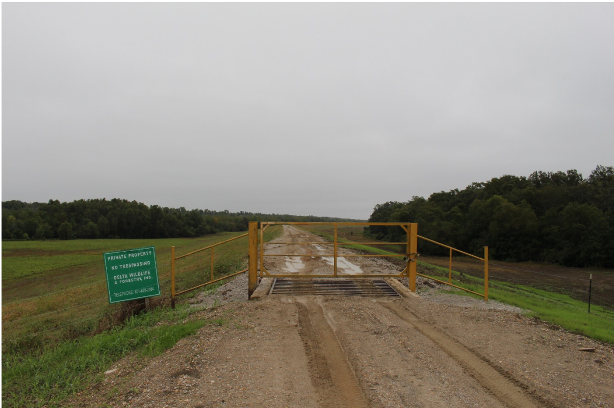
The Mainline Levee just outside of the proposed location for the new pumps project
