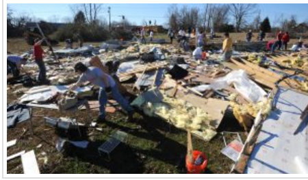
University of Mississippi staff and ROTC students help clean up damage from a February 2008 tornado that hit Oxford. The storms cause severe damage, so everyone should be prepared to act quickly when one strikes. Photo by Robert Jordan/Ole Miss Digital Imaging Services
