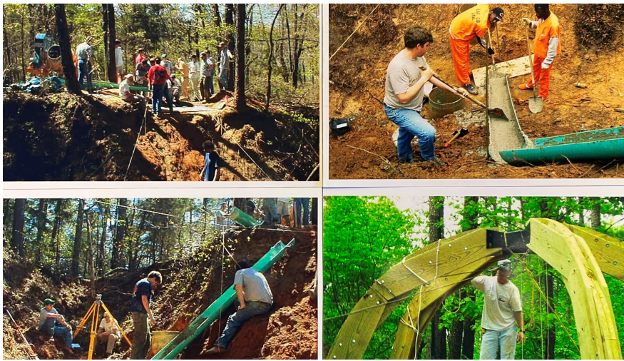
Various phases of construction of the Ladybug Bridge in 2003. Submitted photos
