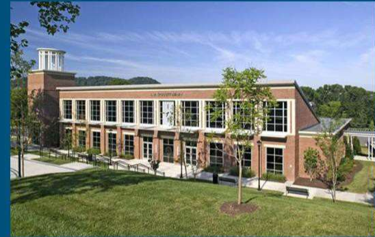
Fig. 15. tuckhinton.com, Franklin Road Academy.
