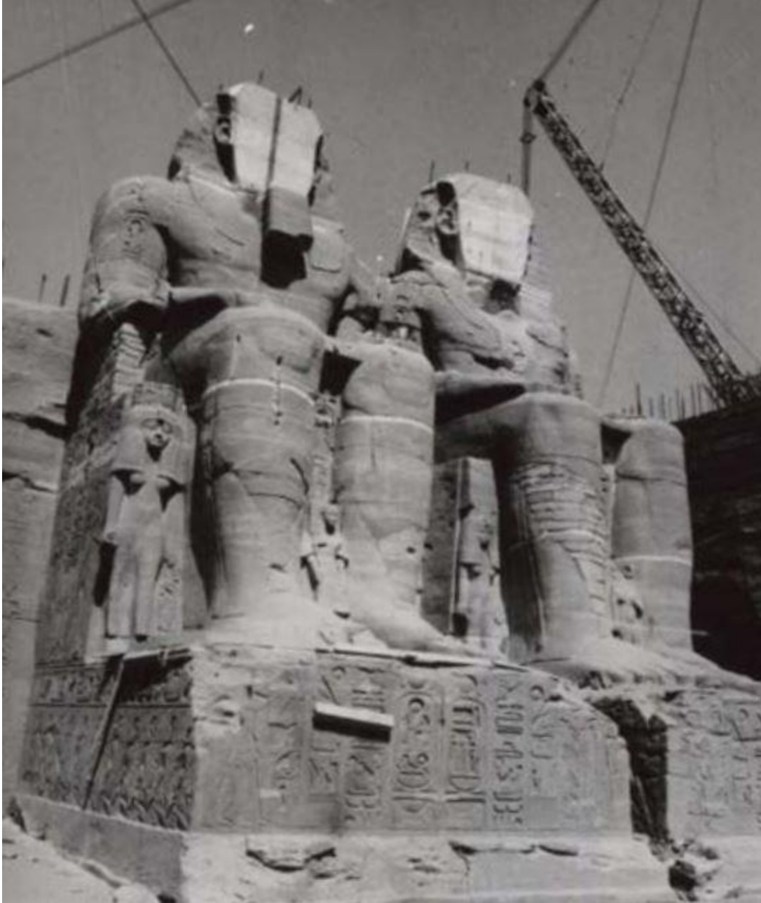
Figure 6, Dismantling Monuments at Abu Simbel, UNESCO
